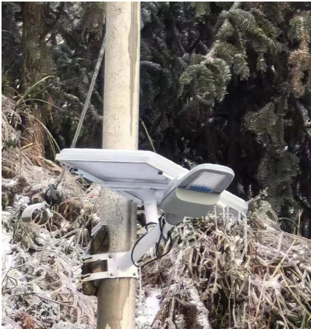
In harsh winter conditions, single-sided charging solar panels: the front was covered with snow, it won't charge.
