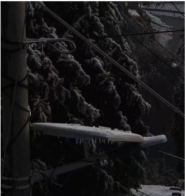
Single-side charging solar energy during the winter the daytime is covered with snow and cannot be recharged by the sun. It can't light up at night.
